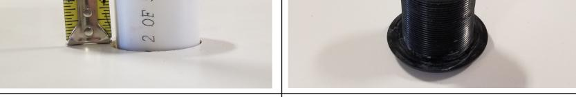
1. Use 1.5" PVC to supply water to the bowl. Cut PVC leaving 1in protruding above the surface where the bowl will be mounted.
