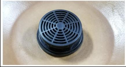
8. Thread in the diffuser to the female threads of the flange. Hand tighten.
