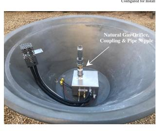
6. Install the Burner Pan. You will need to line up the Opening for the Pilot Burner with the Pilot Burner. You will notice that the hole in the center of the pan (for the pipe nipple coming from the Ignition Control Box) and the opening for the Pilot Burner are much larger than needed. This is done to make it easier to Install the Burner Pan. The large gaps around the pipe nipple and Pilot Burner will be covered with additional parts sent with the Burner Pan in Step 8 below.
