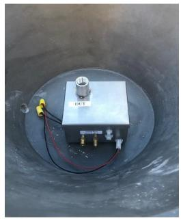
4. On the side of the AWEIS Ignition Control Box there are two brass fittings and two white electrical "Molex" connectors for the Pilot Burner Assembly.
